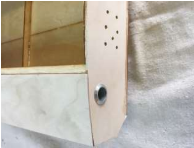
Exhaust outlet. Mount as high as possible.
