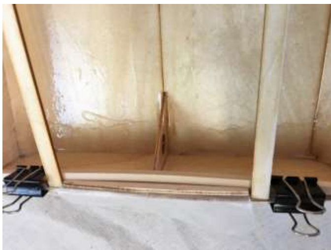
Scrap wood used to hold rear former in place.
